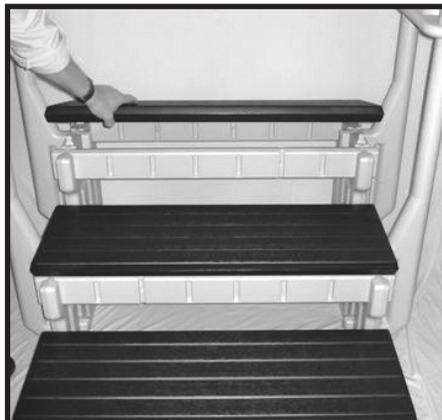
**Step 8:** Install the steps [finished edge out] by placing over the male lugs on the step sidewall and hitting downward with a rubber mallet.
