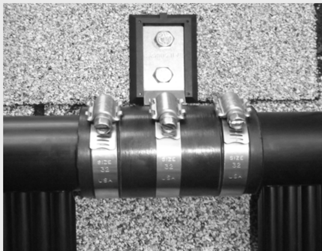
FIGURE 5 Installed Outlet Header Bracket with Hose
