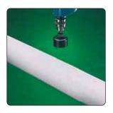
Place the Saddle on a desired location and mark. Remove saddle, drill hole and deburr.
