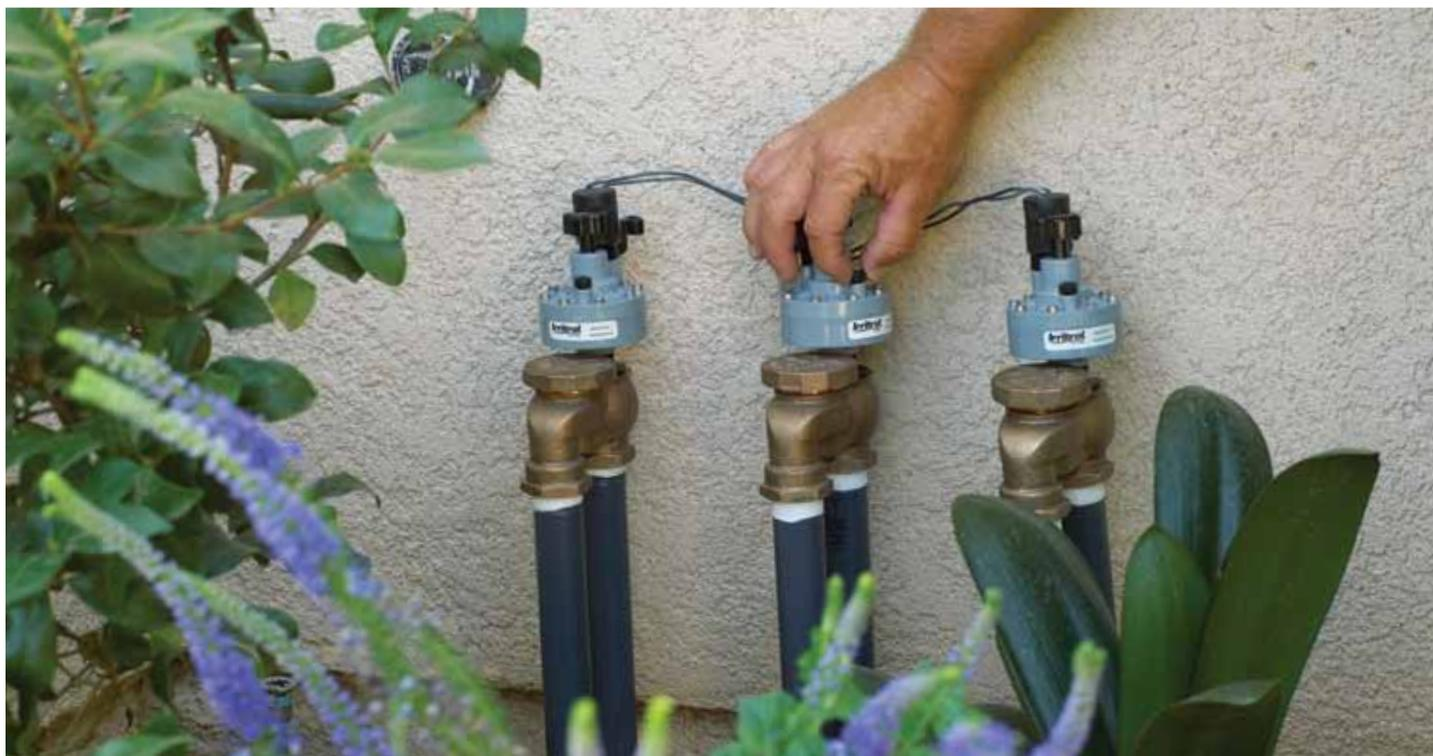
These electric anti-siphon valve adapters feature outstanding durability for consistent, dependable performance in all types of applications. Plus, having all of the internal components captured in a single unit means converting manual valves to electric doesn't get any easier.
