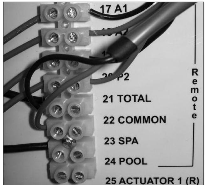
Fig. 11: Heater Wiring Block — Digital Heaters
