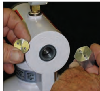
FIGURE 2. Remove security cap with the spanner tool.
